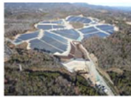
Extra high voltage power plant in Ibaraki
