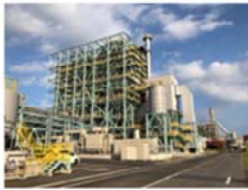
Ichihara Biomass Power Plant
