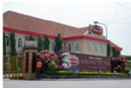
Acecook Vietnam Joint Stock Company's Hung Yen plant
