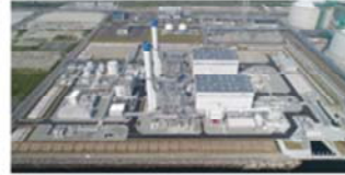
Fukushima Natural Gas Power Plant
