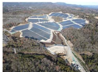
Extra high voltage power plant in Ibaraki
