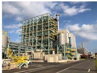
Ichihara Biomass Power Plant
