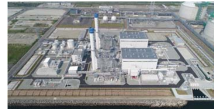
Fukushima Natural Gas Power Plant
