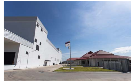
Spiber's structural protein production plant
