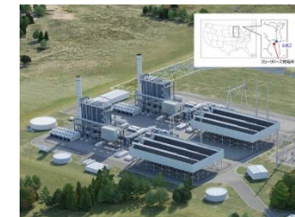
Three Rivers Natural Gas Power Plant
