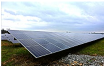
Brighter Future Solar Power Generation
