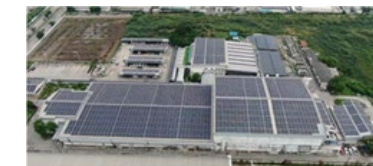
Installation of rooftops at local semiconductor manufacturers' plants
