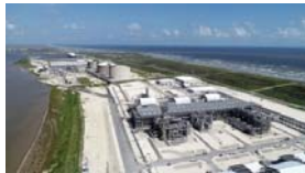
Train 1 of liquefaction facilities in Freeport LNG project (Courtesy of Freeport LNG Development, L.P.)
