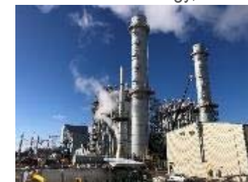
Fairview natural gas-fired thermal power plant in USA
