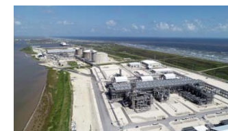
Train 1 of liquefaction equipment in Freeport LNG project (Courtesy of Freeport LNG Development, L.P.)
