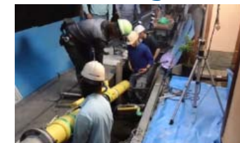
Solving ageing pipe issues
