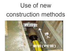
Use of new construction methods The insertion method whereby new PE pipes are inserted into old pipes
