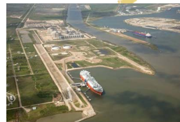
Photograph courtesy of Freeport LNG Development L.P.
