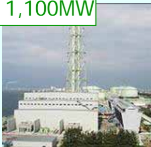
Semboku Power Plant
