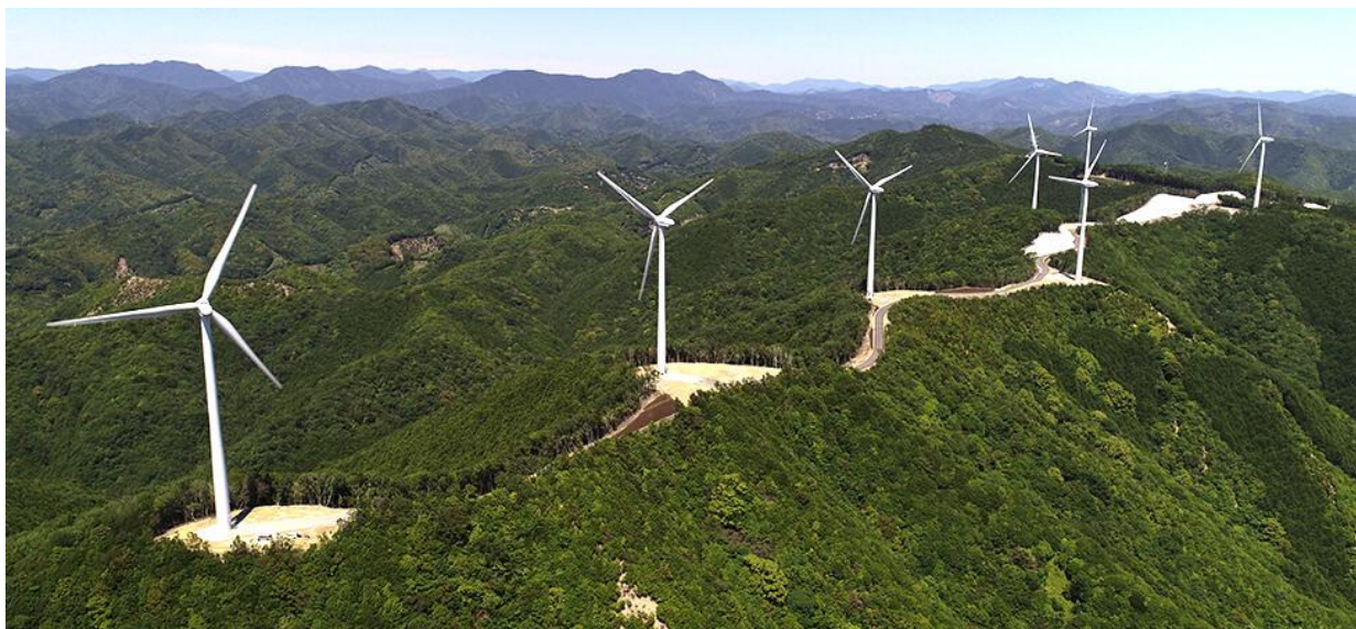
Figure-1 Inami Wind Power Plant
