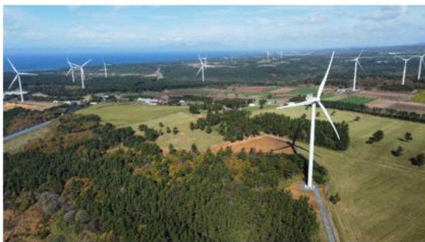
Figure-4 Yokohama Town Wind Farm
