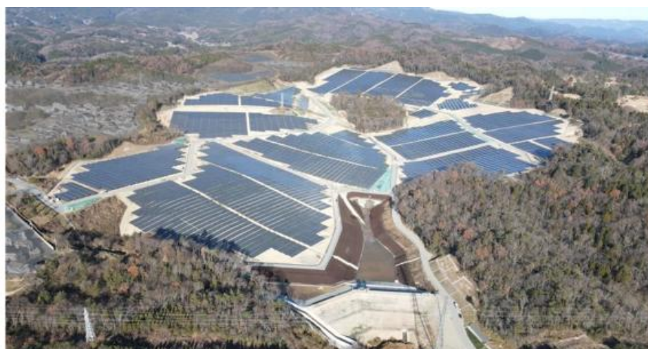
Figure-6 Isohara Extra-high Power Plant
