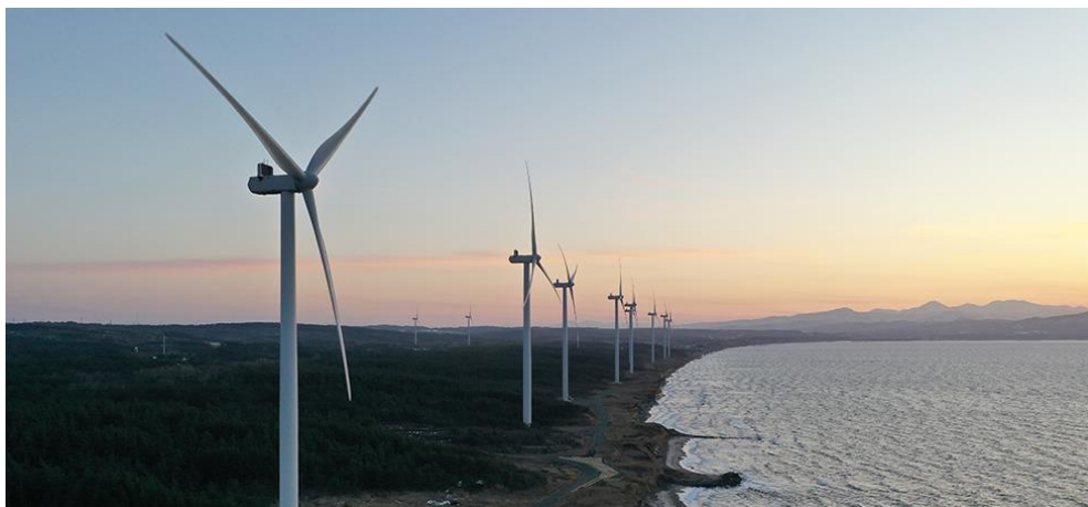
Figure-4 Noheji Mutsu Bay Wind Farm
