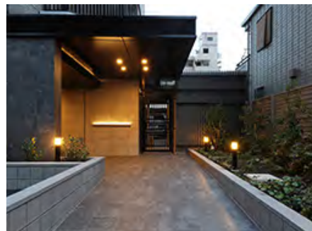
Scenes Tennoji-Karasugatsuji (Completed in March 2025)
