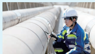
Regular inspection of gas pipes on bridges
