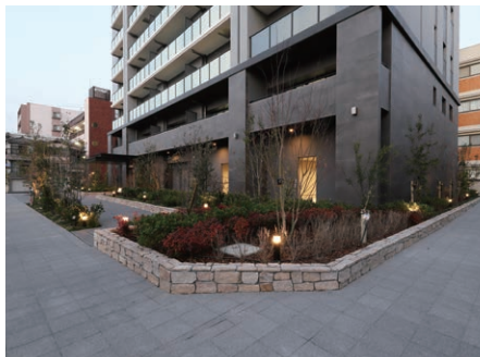
Scenes Midosuji-Abiko (Completed in January 2026)
