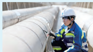
Regular inspection of gas pipes on bridges
