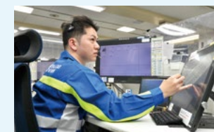
Central Control Room (emergency call reception)
