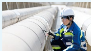
Regular inspection of gas pipes on bridges
