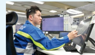
Central Control Room (emergency call reception)
