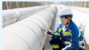
Regular inspection of gas pipes on bridges
