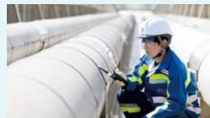
Regular inspection of gas pipes on bridges
