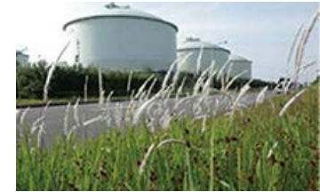
At Senboku LNG Terminal: Green belt planted with Cogon Grass
