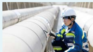
Regular inspection of gas pipes on bridges
