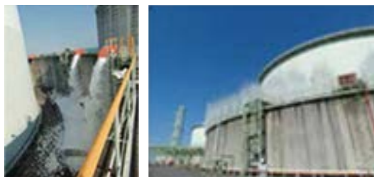
High-expansion foam discharge and water curtain facilities along the dike around an LNG tank
