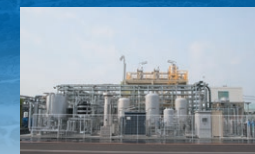
Methanation demonstration facility at the Osaka/Kansai Expo
