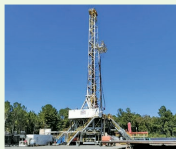
Well drilling site
