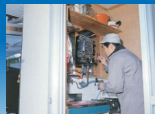
Winter equipment maintenance work
