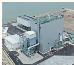
Wakayama Gobo Biomass Power Plant
