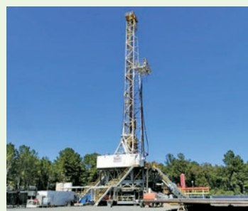
Well drilling site
