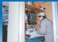
Winter equipment maintenance work
