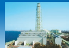
Senboku Natural Gas Power Plant
