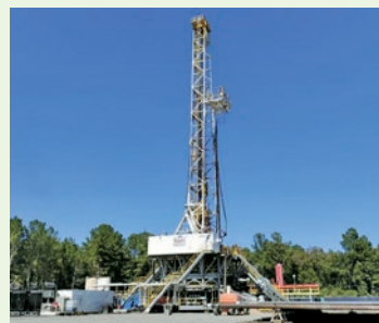
Well drilling site
