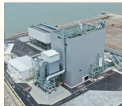
Wakayama Gobo Biomass Power Plant
