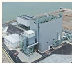
Wakayama Gobo Biomass Power Plant
