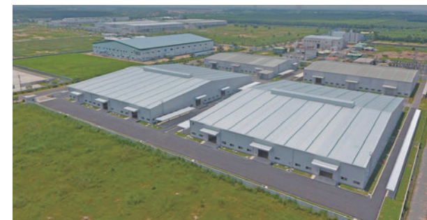
■ Part of Long Duc Industrial Park
