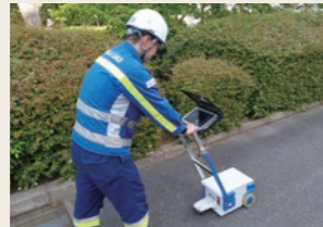
Gas pipes survey using a radar locator
