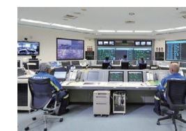
Central control rooms at LNG terminals carry out around-the-clock monitoring and operation of all processes.
