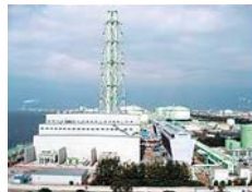
Senboku Natural Gas Power Plant
