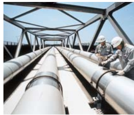
Regular inspection of gas pipes on bridges
