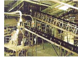
Crushing process during the recycling of excavated soil
