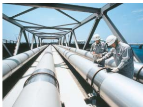
Regular inspection of gas pipes on bridges
