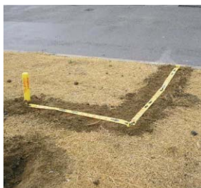
Indication of location of underground gas pipe
