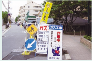
Gas piping work site with Children's Emergency Call signposted
