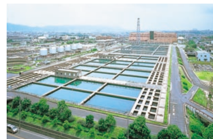
Murano Osaka prefectural water filtration plant
