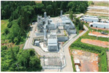
Exterior of the methanation pilot facility (Niigata Prefecture) where we undertake joint demonstration operations with INPEX CORPORATION (Photo courtesy of INPEX CORPORATION)
