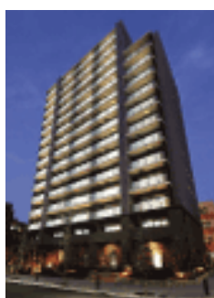
Urbanex Higashiameda (Osaka Prefecture)
