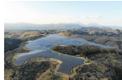
Oita Solar Power Plant (Oita Prefecture)
