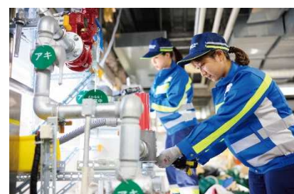
Safety inspection at a supply facility
