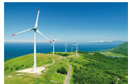
Shiribetsu Wind Power Plant (Hokkaido Prefecture)
