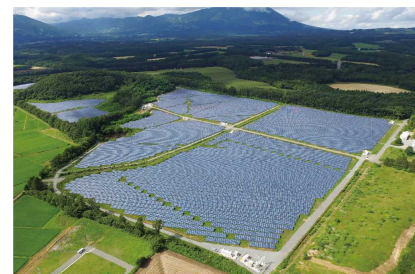
Shizukuishi Solar Power Plant (Iwate Prefecture)
