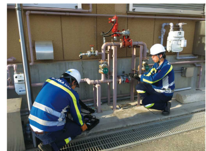
Inspecting the gas supply equipment (emergency shut-off valves)
