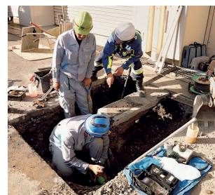
Restoration activities (repairing a gas pipeline)
