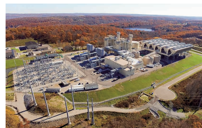
CPV Towantic Energy Center (Connecticut, US)
