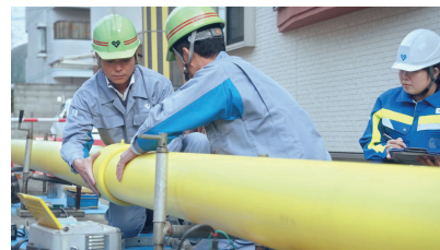
Preparing to bury an earthquake-resistant gas pipeline made of polyethylene
