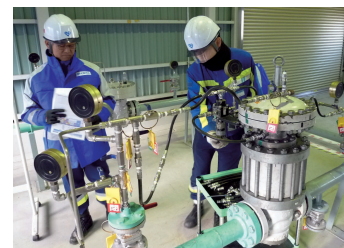
Operational training on gas supply equipment
