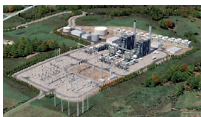
Fairview Natural Gas-Fired Power Plant (Image of completed plant)
