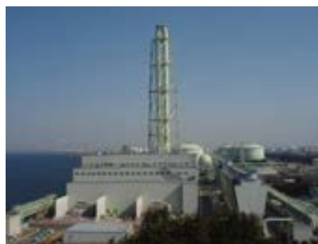
Senboku Natural Gas Power Plant (Osaka Prefecture)
