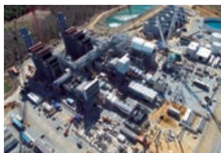
St. Charles Energy Center Natural Gas-Fired Power Plant (under construction)
