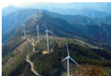
Hayama Wind Farm Power Plant (Kochi Prefecture)
