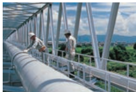
Safety inspection on a bridge pipeline
