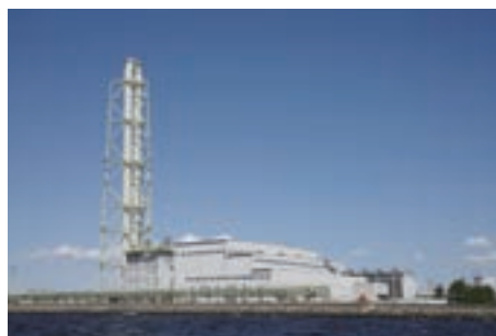
Semboku Natural Gas Power Plant (Osaka Prefecture)
