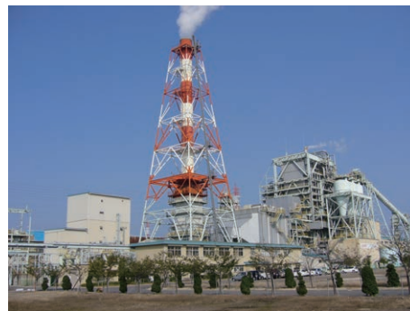
Nagoya Power Plant (coal-fired thermal power plant)
