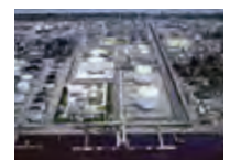
Senboku Plant at start of operations (Osaka Prefecture)
