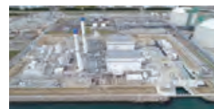
Overall view of the power plant
