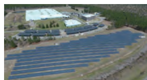
Solar power plant developed and constructed by SolAmerica Energy, LLC in USA Courtesy of SolAmerica Energy, LLC
