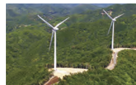
Inami Wind Power Plant
