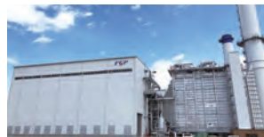
Appearance of Unit 1 (Photo taken on-site: current as of April 2020)
