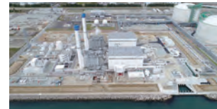
Overall view of the power plant
