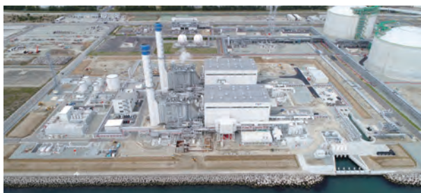
Fukushima Natural Gas Power Plant
