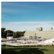
Michigan Power Natural Gas-Fired Thermal Power Plant in the United States
