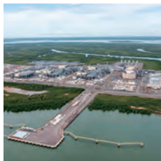
Ichthys LNG Project in Australia Courtesy of INPEX CORPORATION
