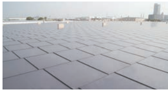
Torishima Solar Power Plant
