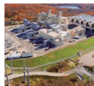
Towantic natural gas-fired thermal power plant
