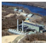
Kleen Energy natural gas-fired thermal power plant
